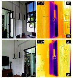
Palo Alto, CA - July 2015 Meeting room wall ndivert panels at **Clarum Hon u**s passive office. Two Ray Magic Gyptone radiant panels installed on the wall next to the door (Gyptone Big Quattro 41 by Saint-Gobain). The radiant panels are in cooling mode with surface temperature at about 57F. • Messana Radiant Cooling
