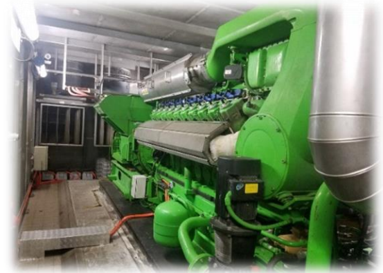
Combined Heat and Power Generator
